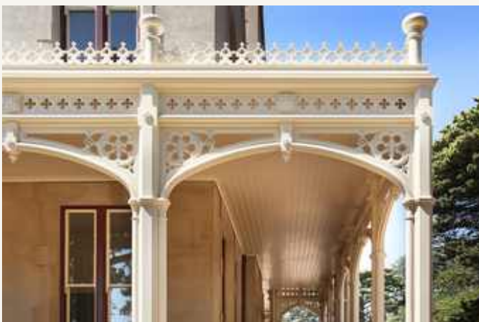
AFTER — REPRODUCED AND REINSTATED IN TIMBER
