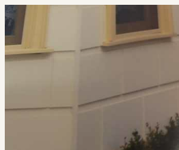
BLOCK WEATHERBOARD — PWB 1
