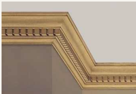
ENRICHED CORNICE, IN SITU — DM 4
