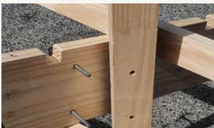
THE JOINT — POST, RAFTER, BATTEN & BEAM
