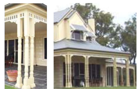
Verandah Posts & Fretwork
