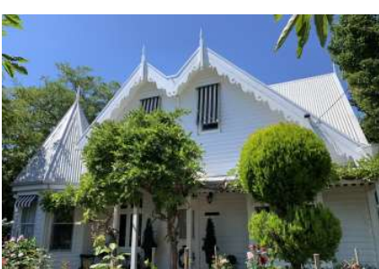
Decorative Barge Boards
